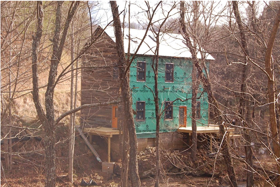
Figure 9: Clark-Miller Mill, northwest corner, view toward the southeast.
