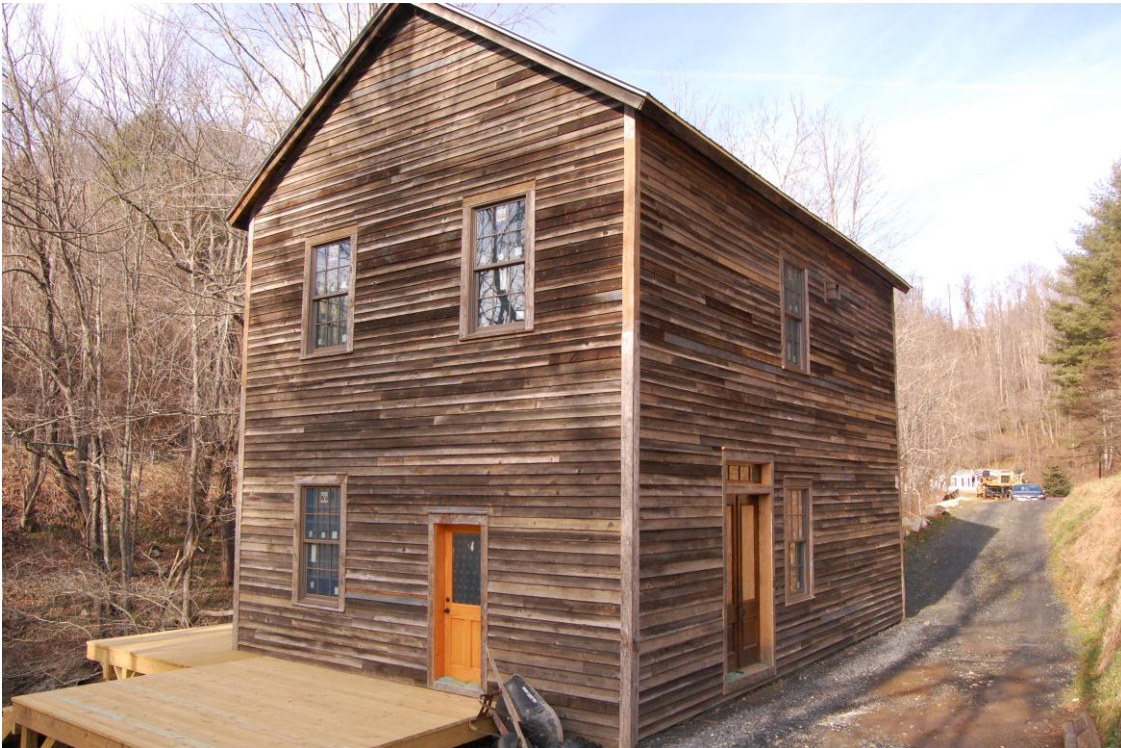
Figure 7: Clark-Miller Mill, southeast corner, view to northwest
