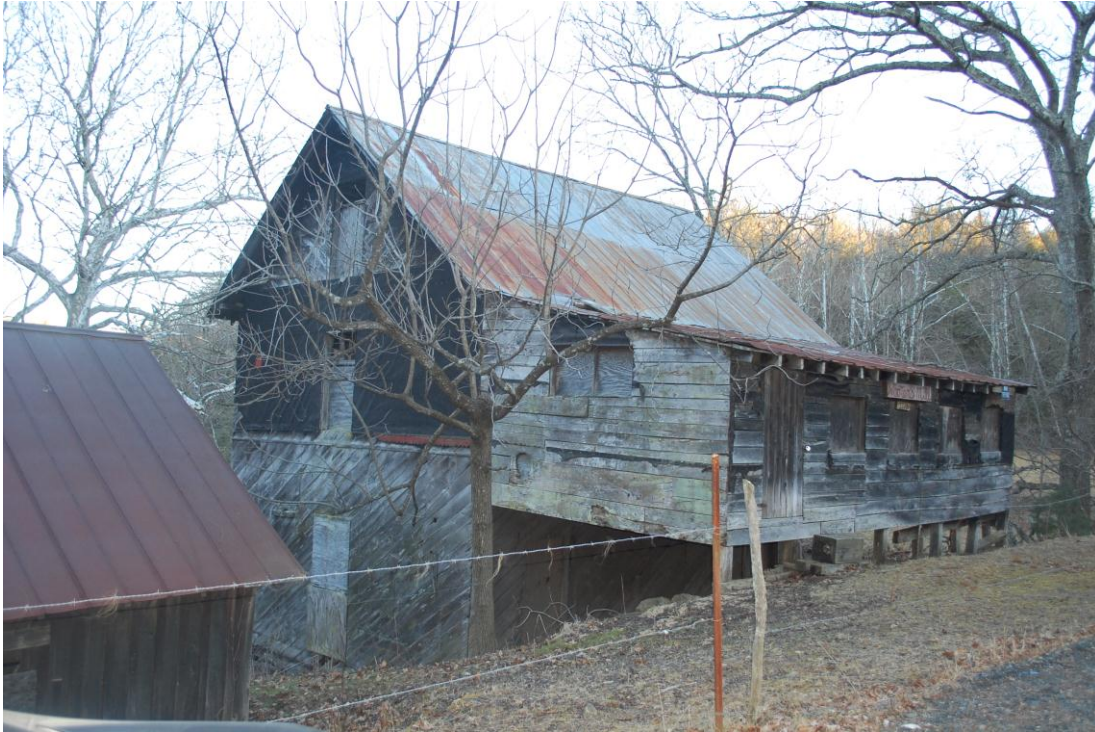
Figure 12: Cockerham Mill (AH 56), view to southeast
