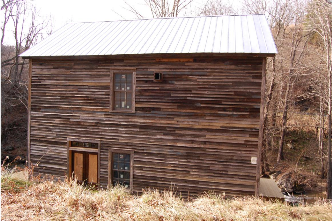
Figure 6: Clark-Miller Mill, south elevation, view to north-northeast
