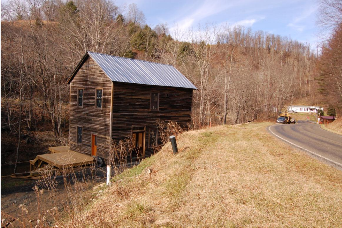
Figure 1: Clark-Miller Mill, 180 Long Branch Road and Bridge No. 61, view to the north-northeast with Long Branch Road (SR 1352) running to the south along Little Horse Creek
