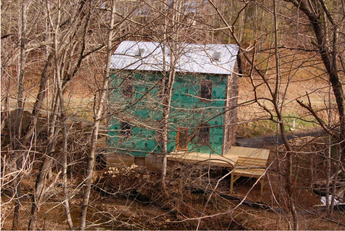
Figure 8: Clark-Miller Mill, north elevation, view to south-southeast
