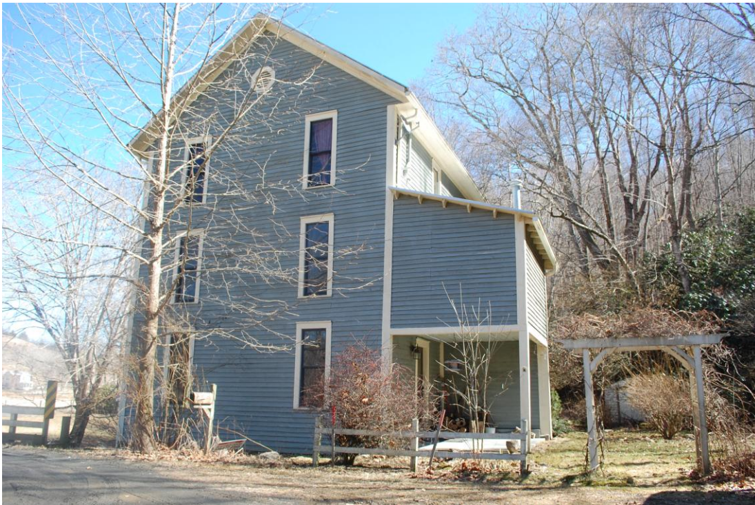
Figure 11: Perkins Flour Mill (AH 59), also known as Helton Roller Mill, view to east
